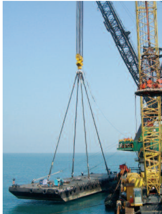
FRANKLIN FLEMISH LOCK slings lifting 1,800-tonne test lift
