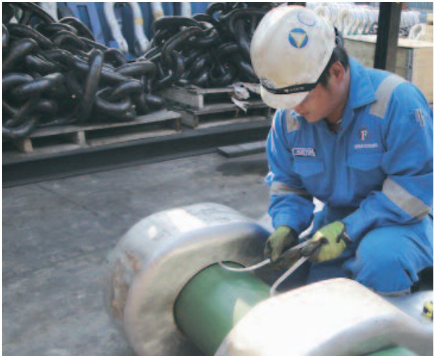
Inspection of Sling Saver Shackles
