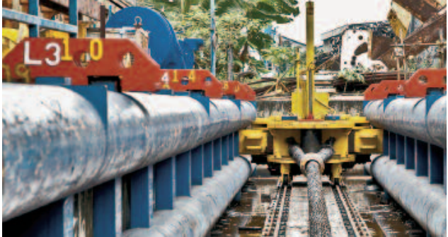
Load Testing of Cable Laid Slings
